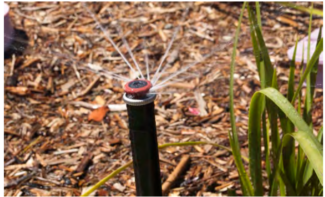
Rotator nozzles throw streams of water with larger water droplets which helps to prevent misting and runoff, but each nozzle still needs to be checked periodically to ensure it is running correctly.
