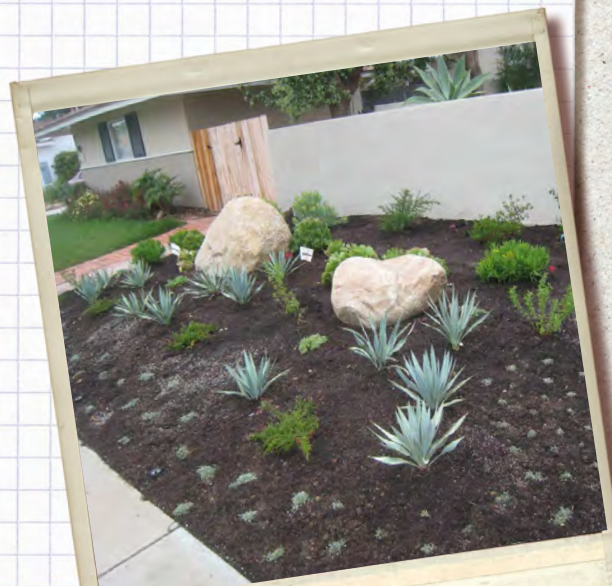
San Diego Residence -Planting Installation-
