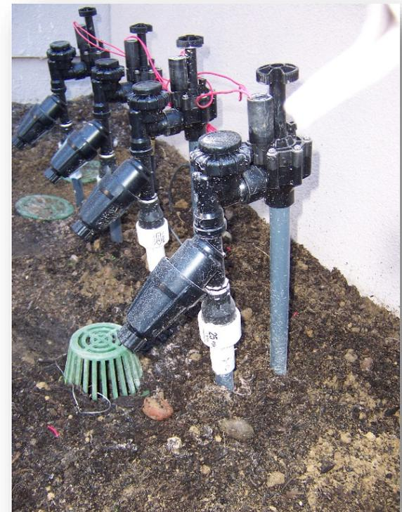
**Low flow zone kit – valve, filter and pressure regulator**
