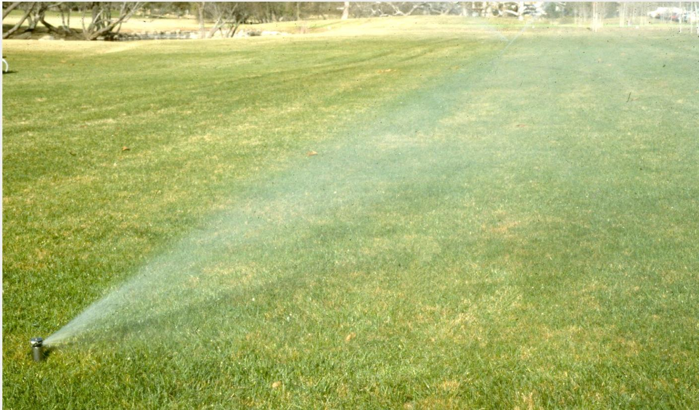
**Rotor stream should fan out and disperse evenly from beginning to end**
